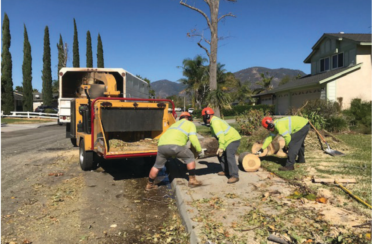
Work completed on La Selle Ave.
